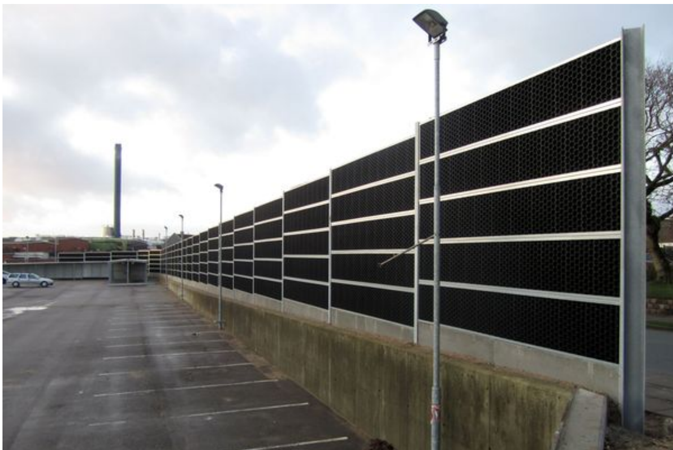
The noise barrier absorbent side showing the cassettes containing acoustic absorbent material of recycled glass fiber. Source: Miljoskarm
